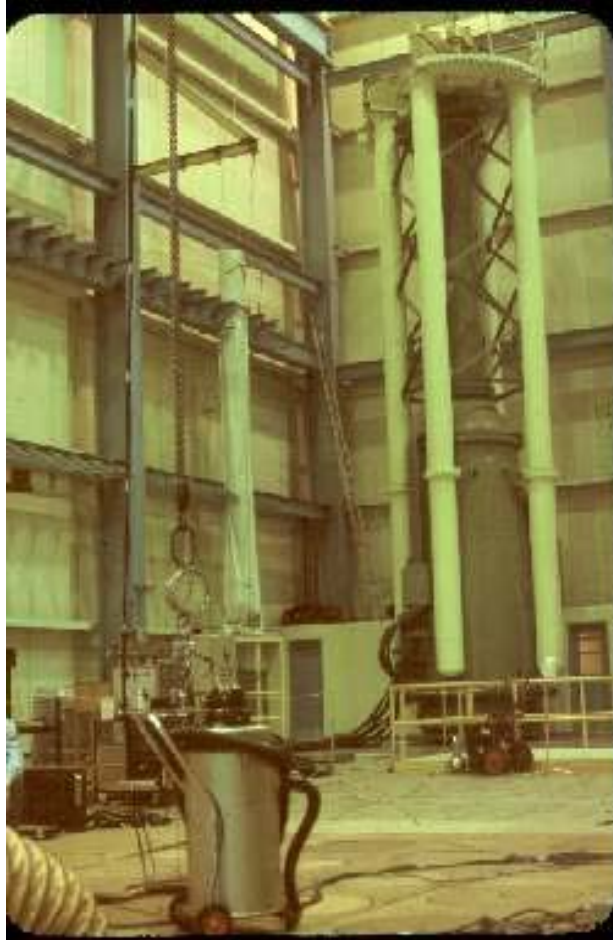
Fig. 4.4. Photograph of Fort St. Vrain refueling machine.
