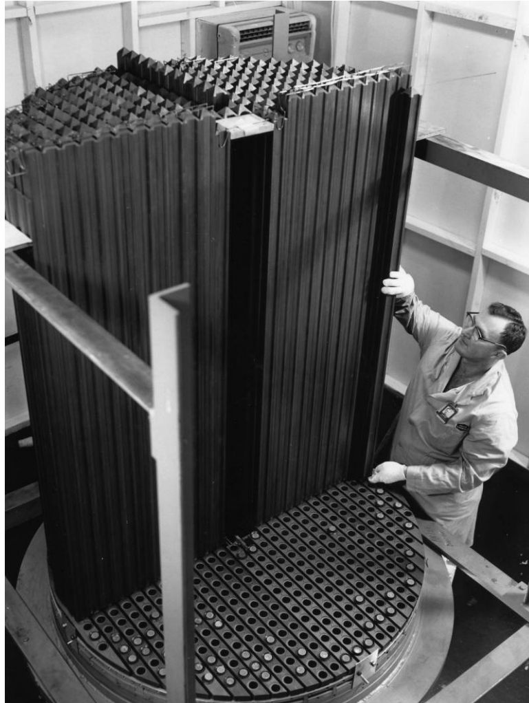
Fig. 23. Graphite core of the MSRE.
