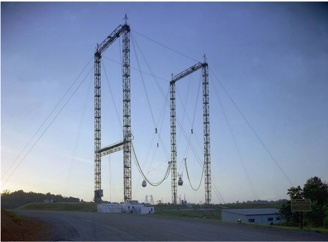
Fig. 41. A reactor and shield suspended at the TSF. (ORNL Photo 50397)
